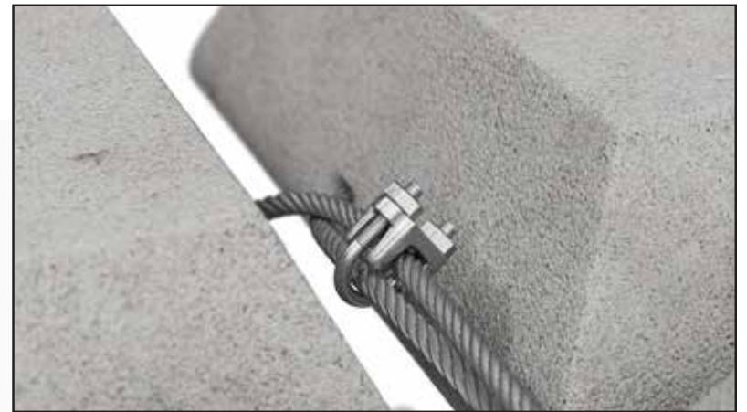
Articulated Concrete Cable Block Mats are joined together with Cable Clamps
